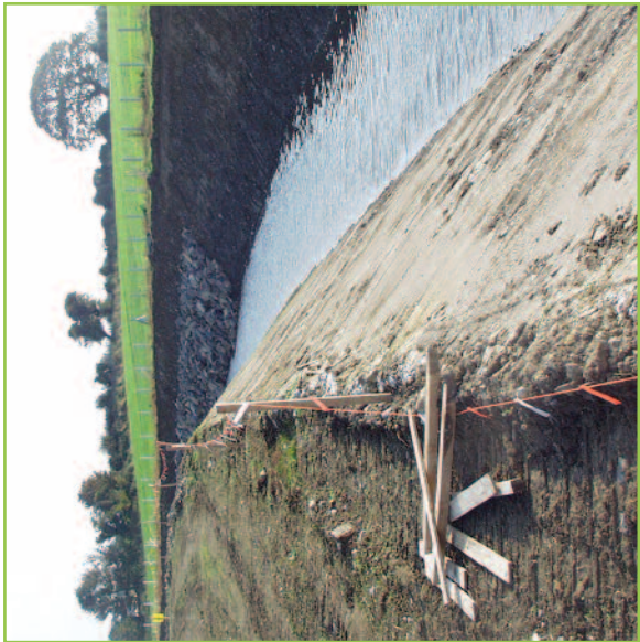
A poor example of a realigned watercourse with a highly uniform trapezoidal profile and flow regime. This limits the ecological potential of the river as well as reducing landscape quality through a "loss of naturalness" within the landscape.
