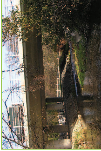
A well designed clear-span bridge retaining the existing river channel with piers set back from the river bank.
