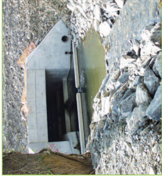
A well designed culvert which has a stepped profile to accommodate fish passage and an outlet pool to allow fish to pass upstream into the first of the steps. The culvert incorporates a cast mammal ledge.
