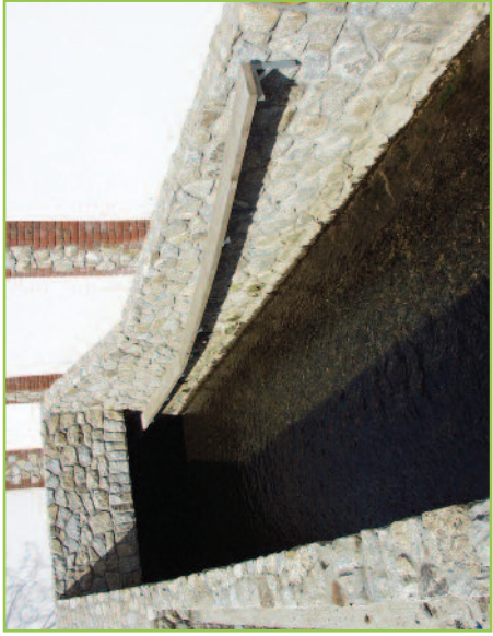
A culvert with an otter ledge attached on brackets. This section of artificial channel has a stonepitched base on which sand and gravel will lodge more readily than concrete.
