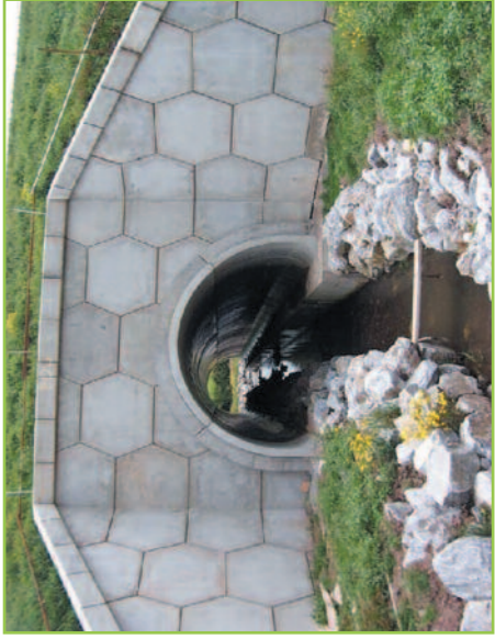
An example of a well designed oversized arched culvert with mammal ledges. The natural bed of this watercourse was maintained.
